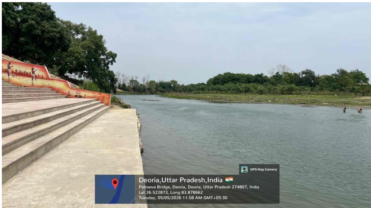
Figure 5: River embankment & RFD works done on Chhoti Gandak River by Flood Work Division, Deoria
