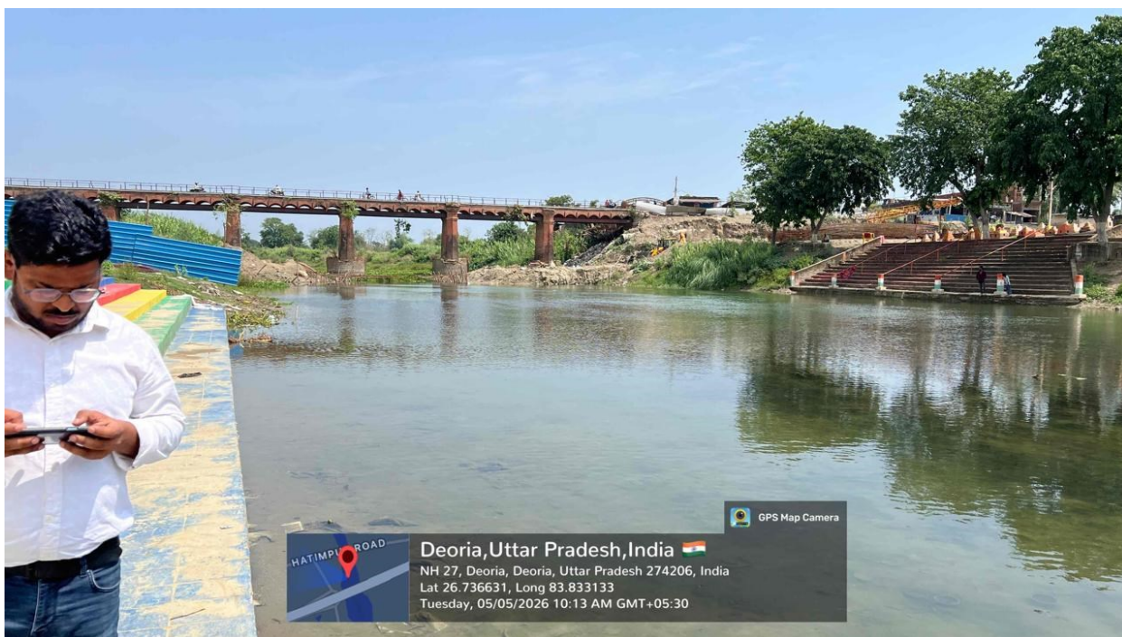
Figure 2: Chhoti Gandak entering in Deoria District at village Bhataulli, Hetimpur & RFD work done by Flood Work Division, Deoria
